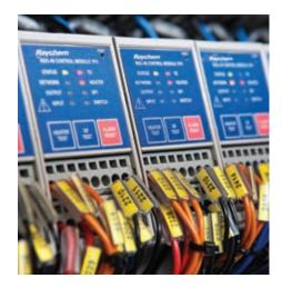
Central control and monitoring systems are typically installed in panels where they provide control and monitoring for several heat-tracing circuits or groups of circuits at the same time. They offer advanced features like measuring ground-fault levels, operating currents and provide a wealth of other maintenance-related information.
